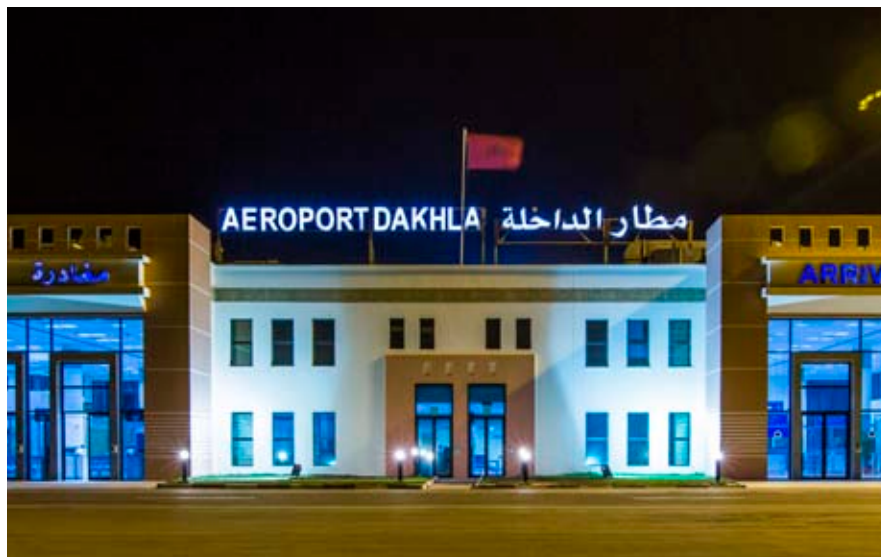
Dakhla Airport, Morocco
